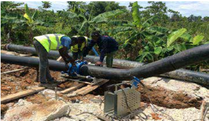
Installation Works at Different sites
